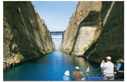
Crossing the Corinth Canal
